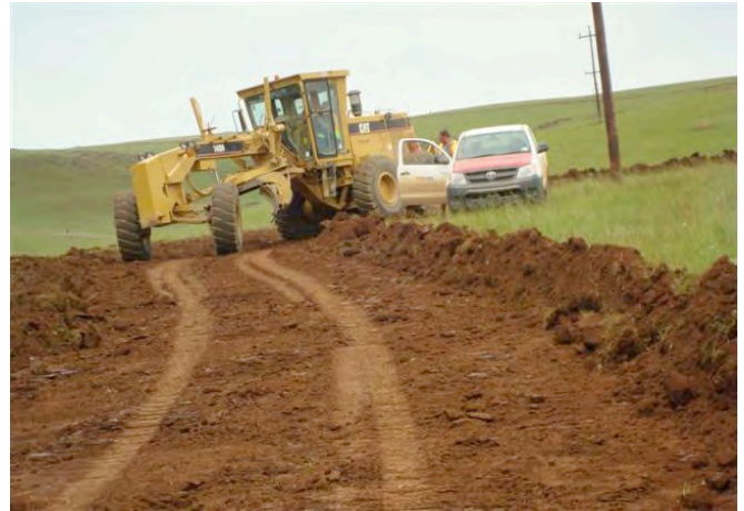
WBHO's Roads Team grading the road to the Umzimvubu Feedlot
